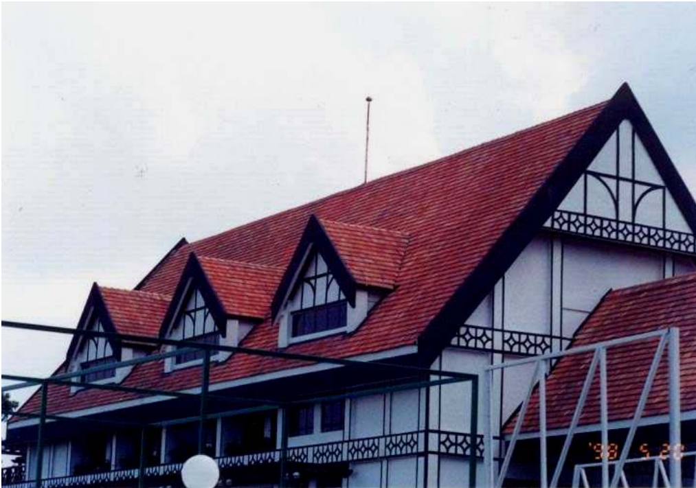
Figure 8: The Dynasphere installed on the roof of the RSC building in 1998.
