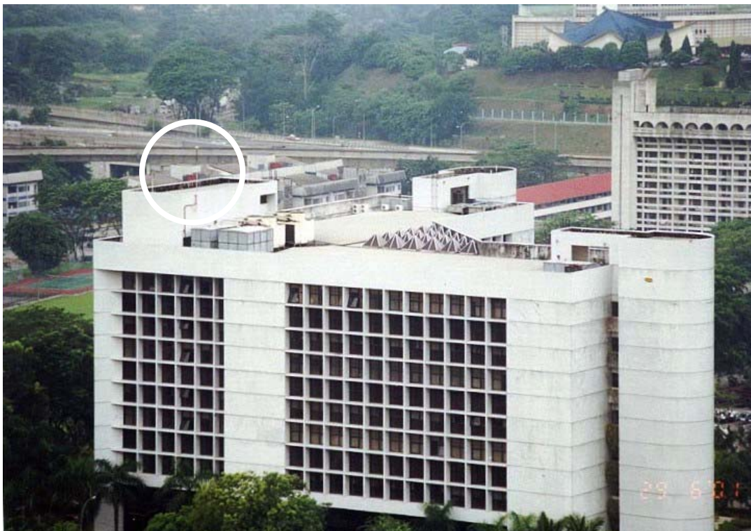
Figure 12: The DCS building photographed from another building which is located to the North-West. The Dynasphere air terminal (circled) was installed at the centre of the building.
