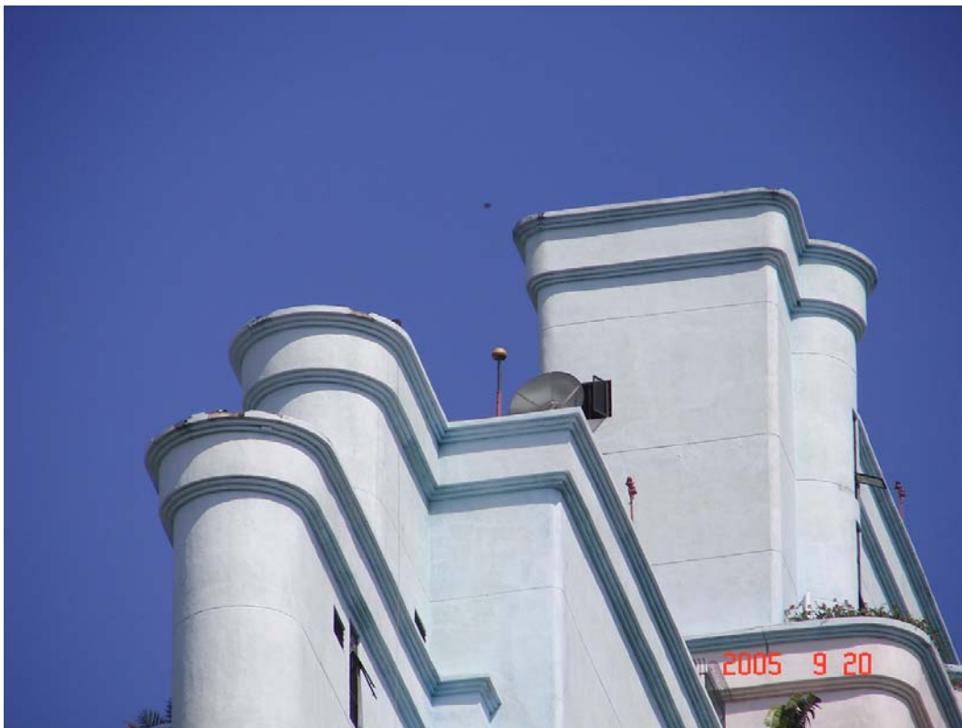
Figure 20: A view of the Villaputri building from a different angle. Since the curved edges had been struck by lightning repeatedly, the claimed existence of the collection volume is doubtful.
