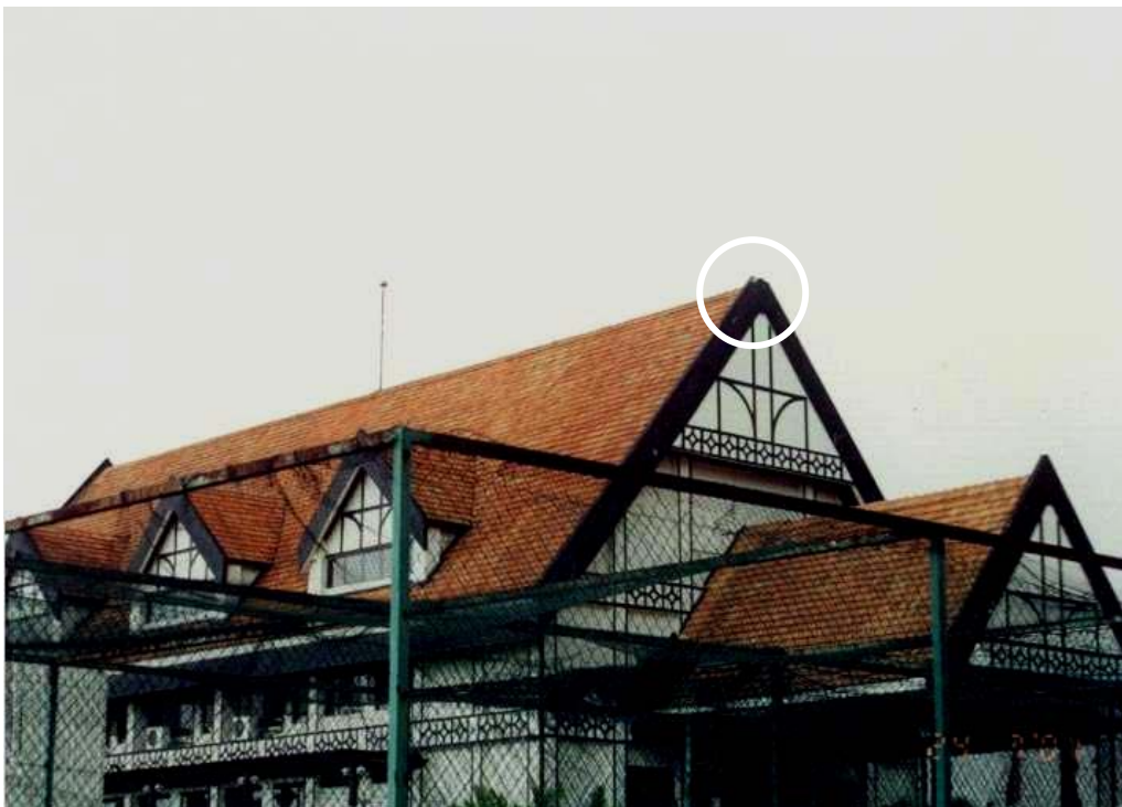
Figure 9: The bypass on the front façade observed in May 2001.
