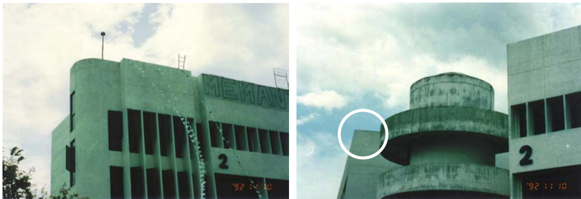
Figure 4: The Dynasphere on Building 2 (left) and the undamaged roof corner of Building 3 (right) taken in 1992.
